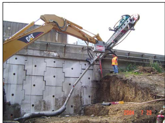
Photo 2 Soil Nail Installation
