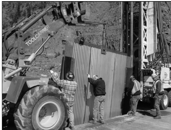
Installing verification “Test Panel” into slot.
