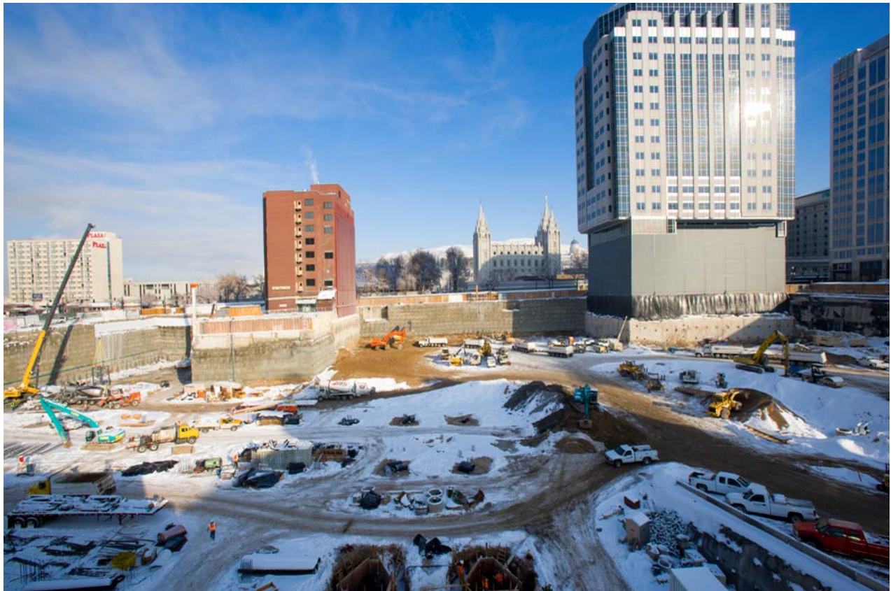
Figure 12. General site view looking north.
