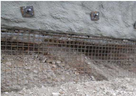
Figure 9. Open coarse cobbly zones (top) and lost ground zones (bottom).
