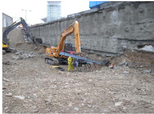
Figure 4 –Concurrent Demolition and Soil Nail Wall Installation.
