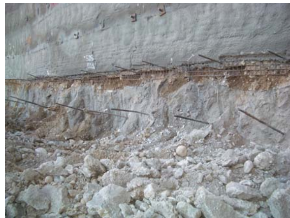
Figure 7 –Jet Grout Wall South Temple Street
