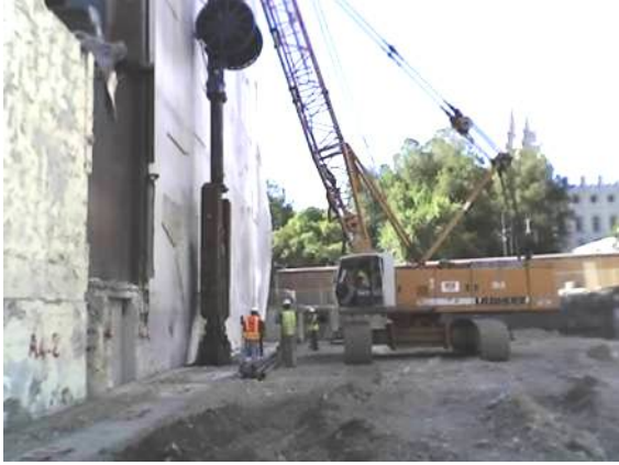
Figure 8 –First Anchored Diaphragm Wall in Salt Lake City June 2007
