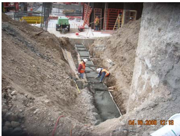
Figure 11. Sequential installation of subsurface struts at west wall of Gateway Tower.
