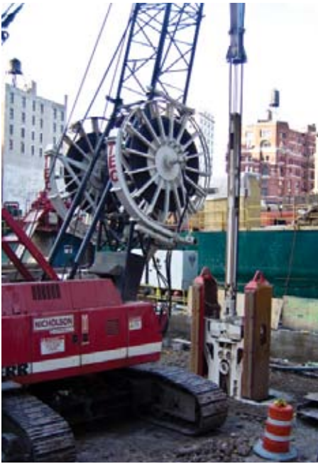
Diaphragm wall excavation (left); Interior steel column with barrette foundation (right)
