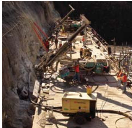
Overview of drill platform and work area (left); Drilling vertical tie-downs (top right); Rigs drilling incline anchors through the dam (bottom right)
