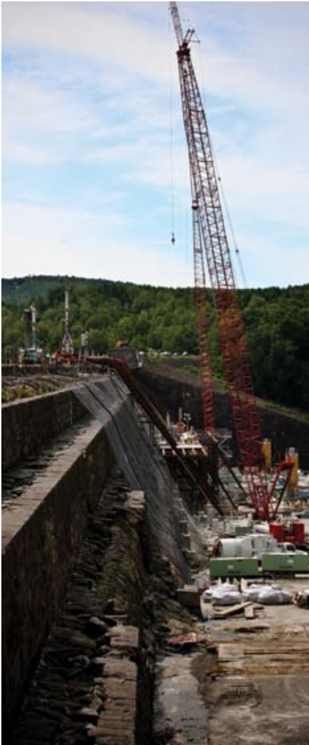
Overview of drill platform and work area (left); Drilling vertical tie-downs (top right); Rigs drilling incline anchors through the dam (bottom right)
