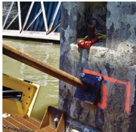
Self contained drilling and grouting support barge (top); Side view of drill platform (bottom left); Close-up view of anchor drilling (bottom right)
