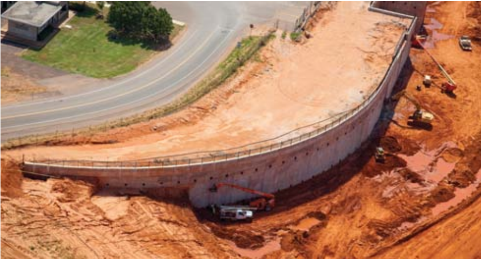
Northern diaphragm wall
