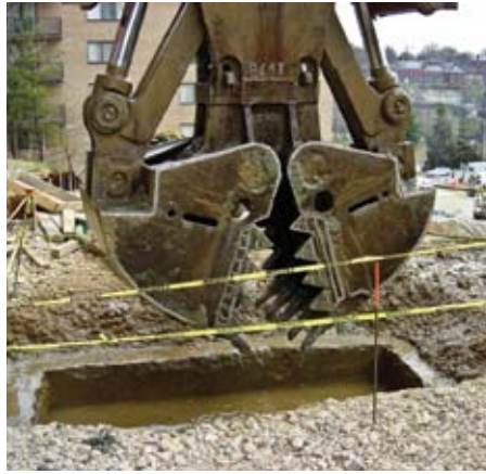
Hydraulic clam shell used for barrette installation
